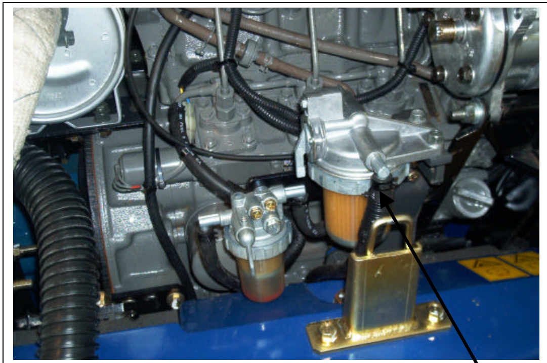
Fuel filters relocated with new bracket installed for smaller filter.
