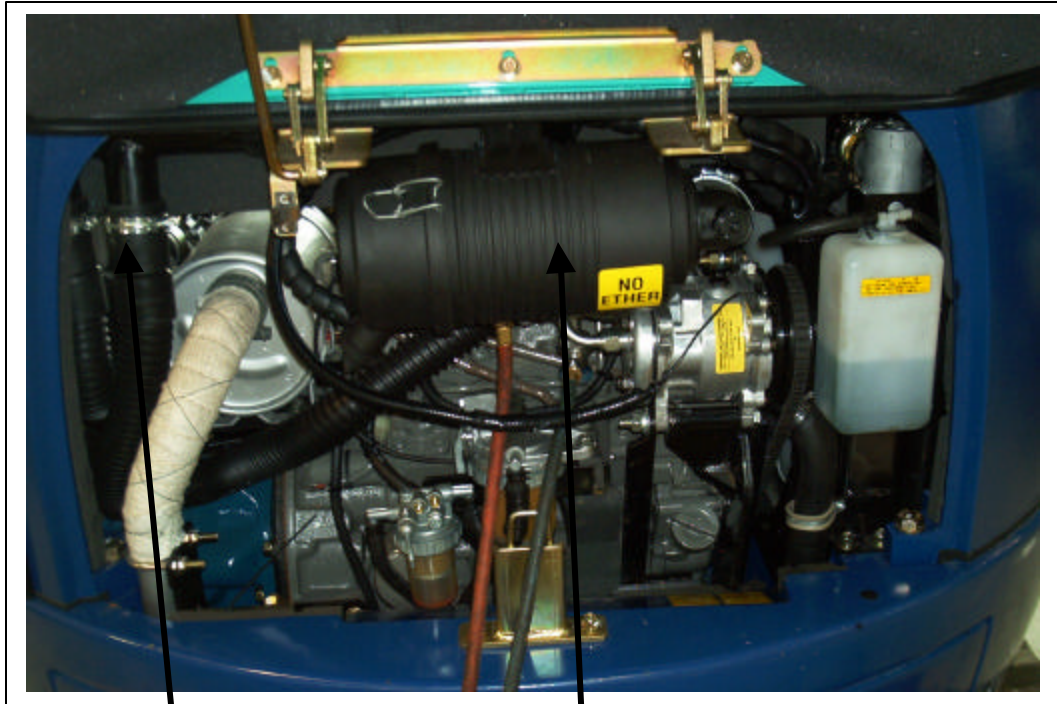
New hose hook up for air intake
